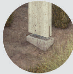
Close up. Foundation
