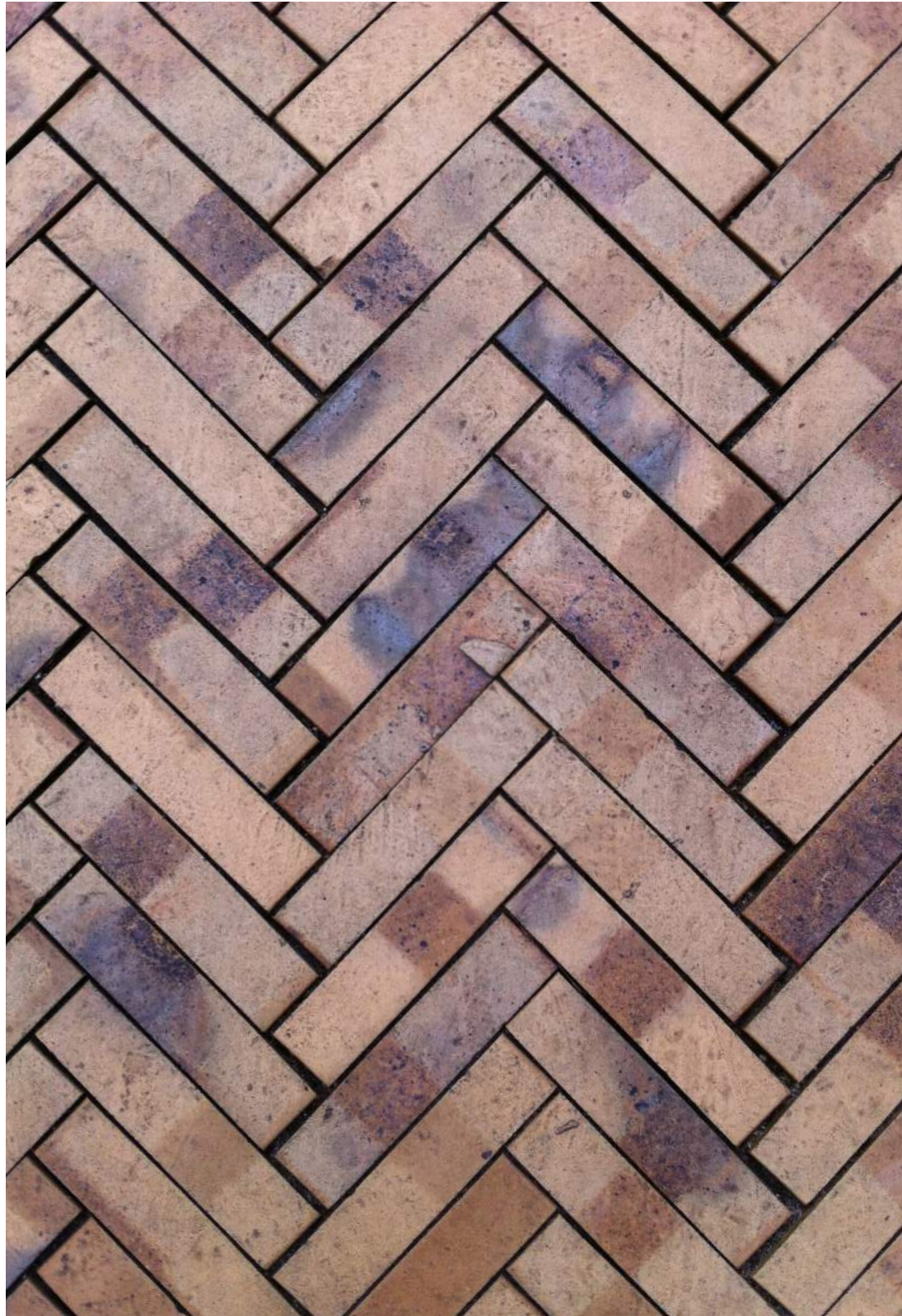
Coal-burned clinker bricks complementing the soft wooden surface.
