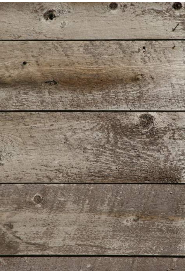
Wooden deck for the twirling bridge.
