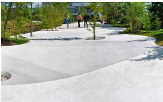
Recycled concrete cast texture.
