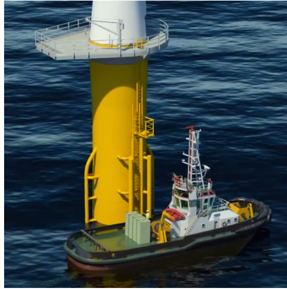
Fig 1.2. Transition piece with visible secondary structures, e.g. boat landing. [COWI, 2010]
