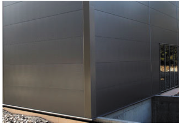
Ill. 48 // Sandwich panel cladding example
