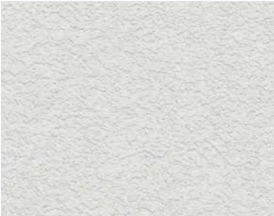
ill. 4.55: Plaster walls
