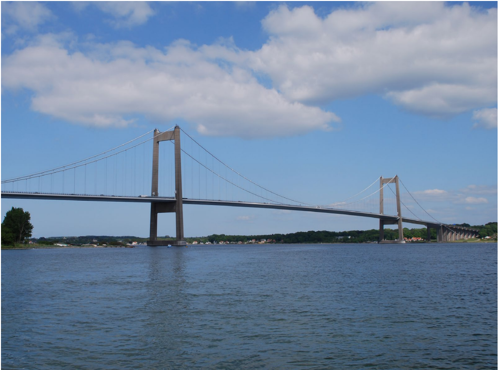
III 39: A view of the Lillebælt bridge
