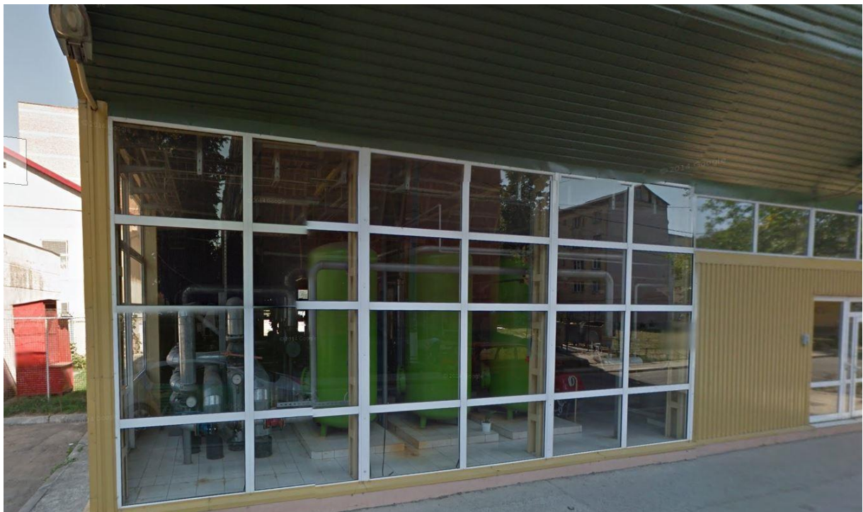
Figure 15 Ferroli industrial size gas boilers (3x2,000kW) (2)
