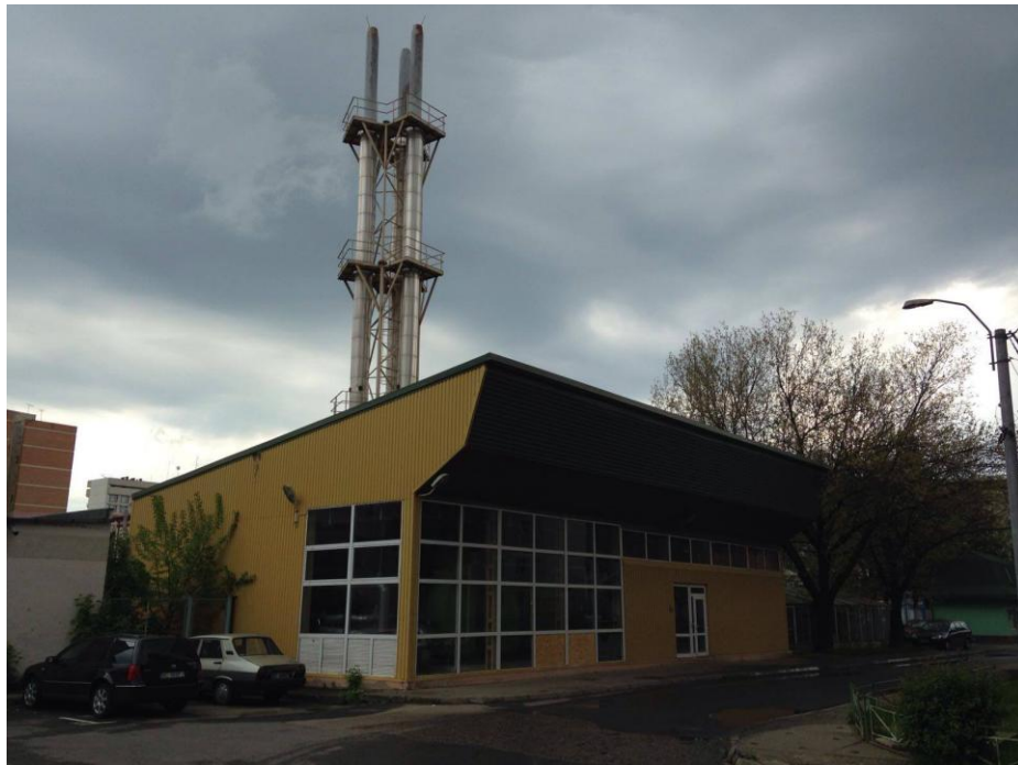
Figure 14 Ferroli industrial size gas boilers (3x2,000kW) (1)
