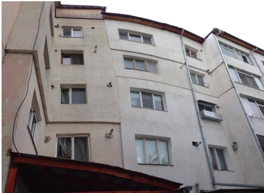
Figure 10 Outside view of the drain pipes (2)
