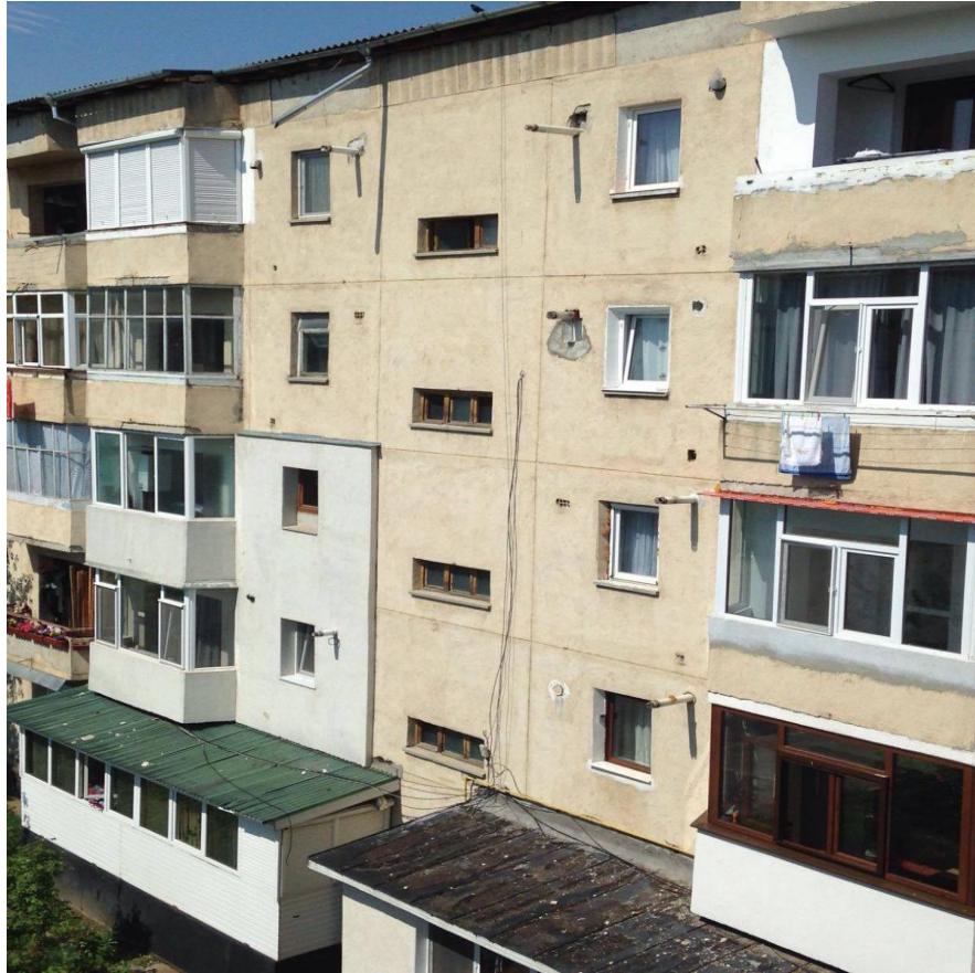
Figure 9 Outside view of the drain pipes (1)
