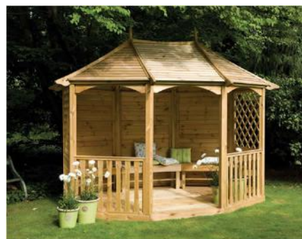
III.88. Wooden shelter protects from wind and rain
