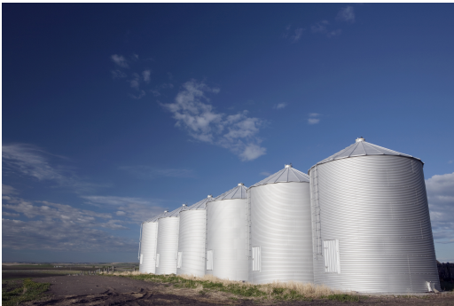
Figure 1.1: Silos made by shells [Thebimhub, 2016].
