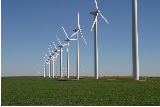
Figure 1.3: Wind turbines [Positronic, 2016].
