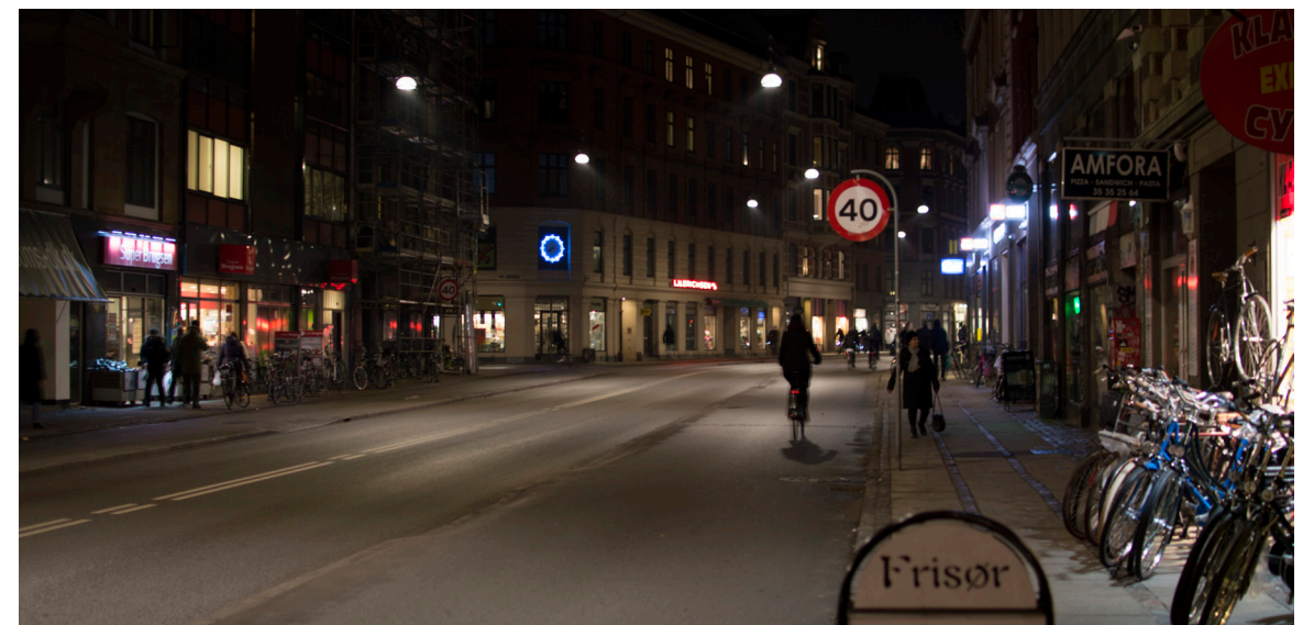
III. 41. A more equal hierarchy doesn't have to require advanced solution. On Nørrebrogade, the use of two rows of wire mounted luminaires instead of one centrally mounted row creates a relatively equal hierarchy across the street's profile, resulting in good overview for all users.
