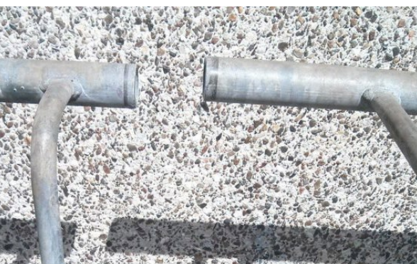
Ill. 32: Example of rack lock cut by a blowtorch.
