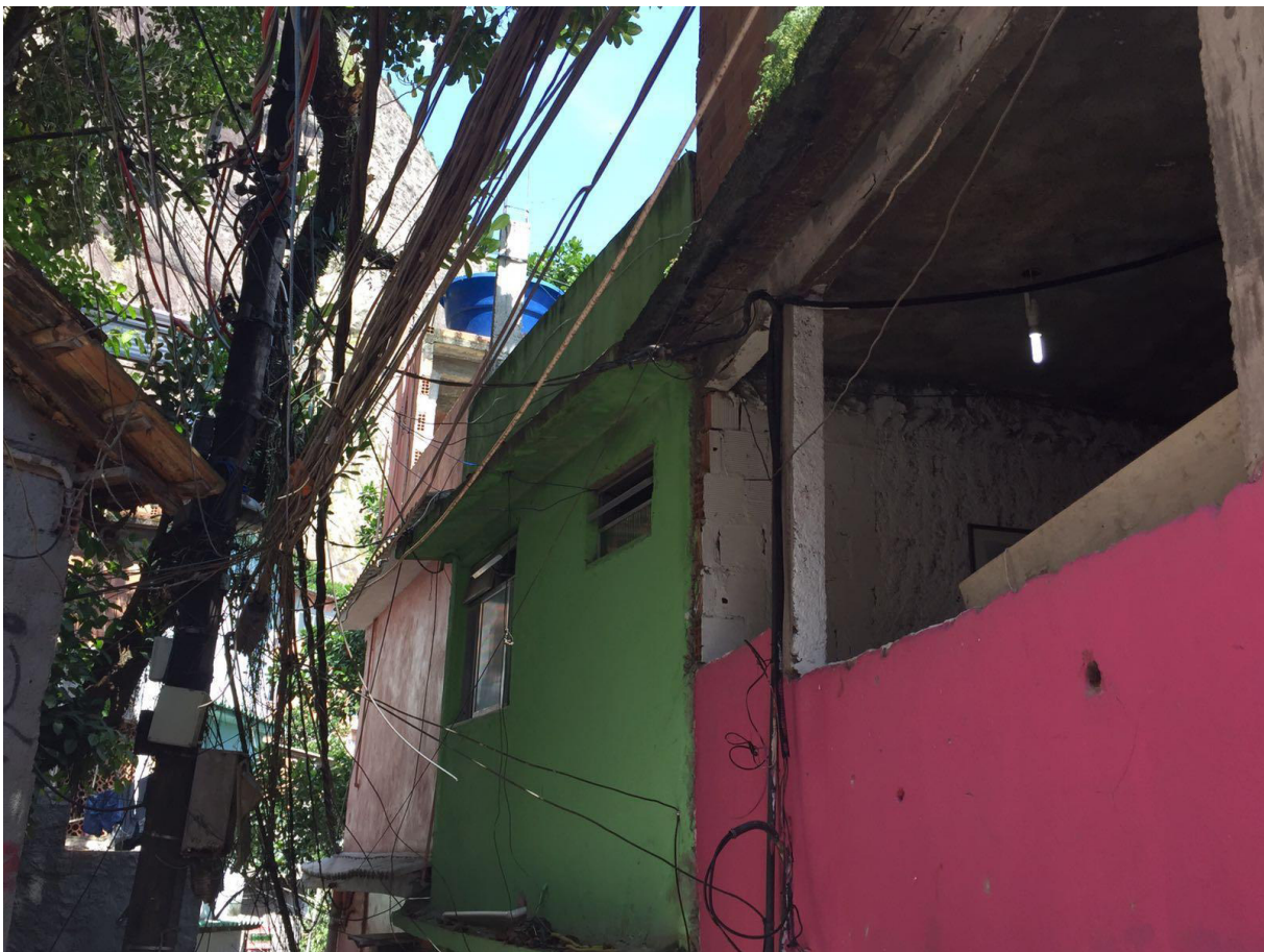
Figure 1: Usage of illegally tap electric wires in Latin America`s biggest favela Rocinha in Rio de Janeiro. (Source: Author photo, (2016)).
