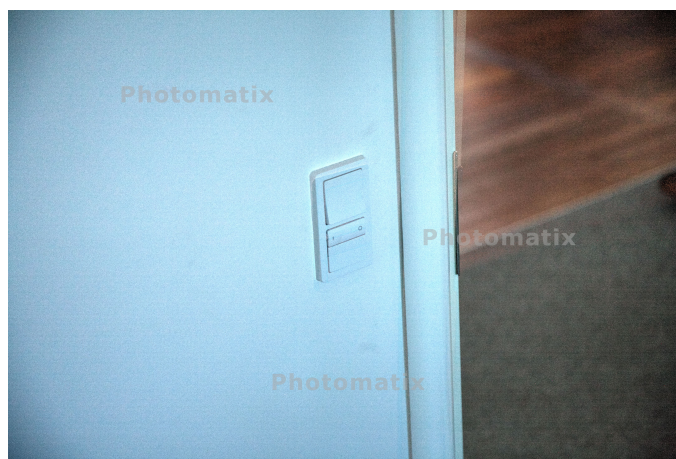
Figure 4.9: One of the controls for the lights in the offices.
