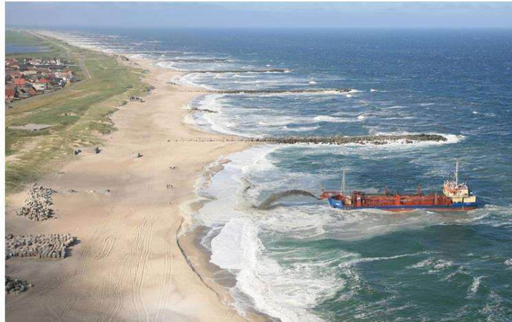
**Figure 1.3:** Protection works along the West coast. Groynes construction and sand nourishment [6]
