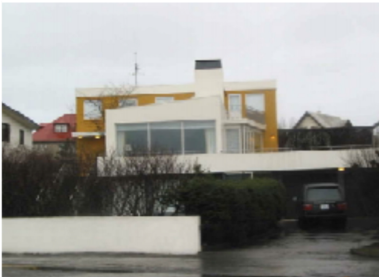
Figure 9: Ægisíða 80, a building well known for its modernist architecture. The north facing side of the house holds the bedrooms (Gylfadóttir, Gunnarsdóttir, & Ármannsson, 2005).
