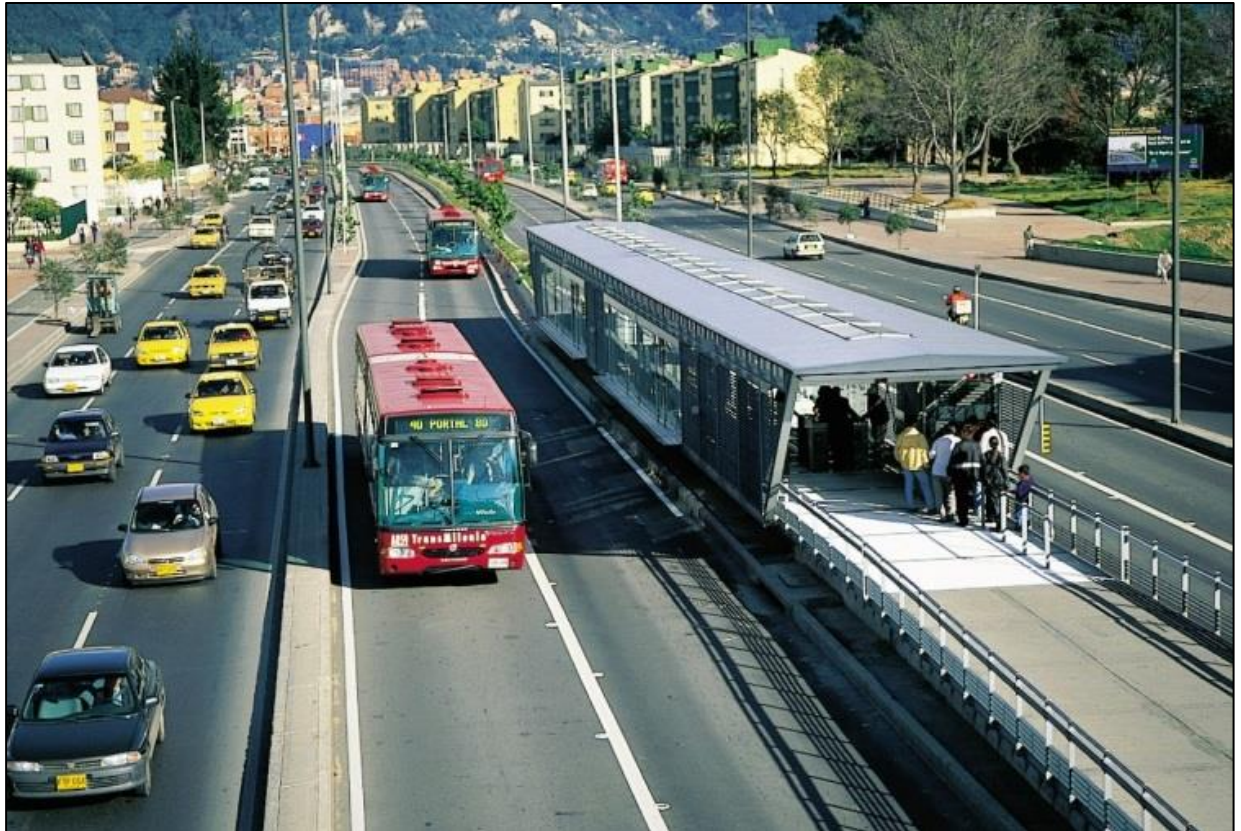
Picture 6. Transmilenio station located between two fast, separated bus lanes. (Martinez, 2013)
