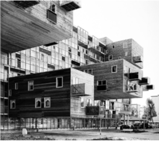
Figure 12 MVRDV going against the principle of legibility by hiding the steel vierendel structure in wood cladding
