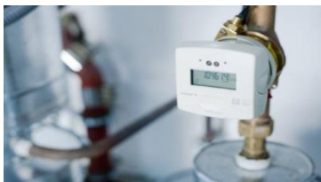
Picture 18-heat meter
