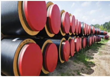
Picture 8-DH pipes on the left
