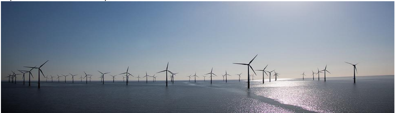
Picture 23-Wind mills in Kriegers Flak, Denmark's to date largest offshore wind farm in the waters between Møn, Southern Sweden and Northern Germany
