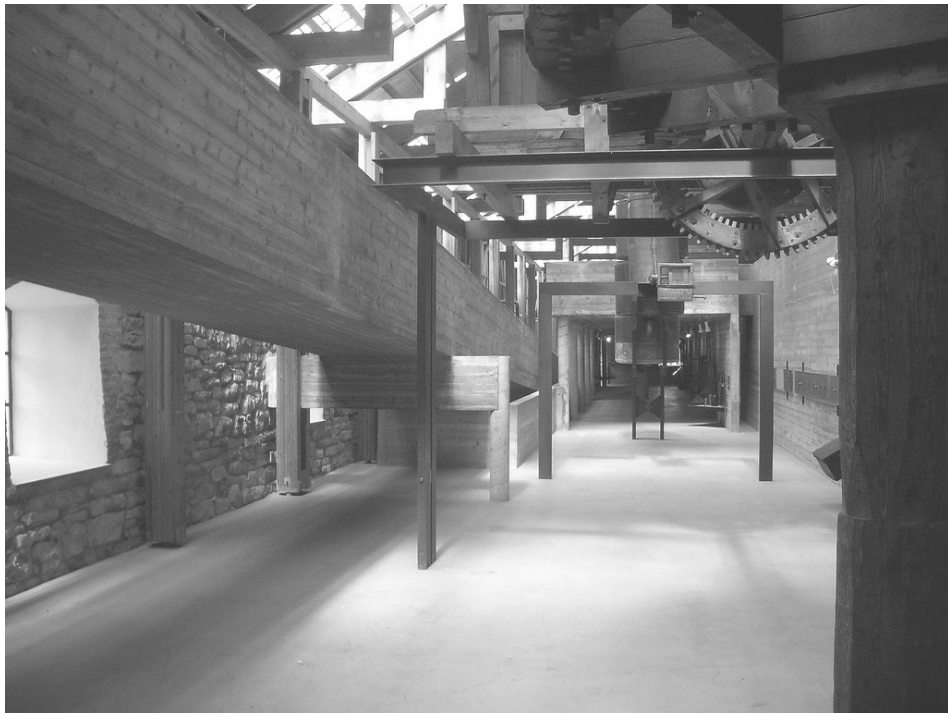
The new elements are gently lifted above the old to show clear separation - 10
