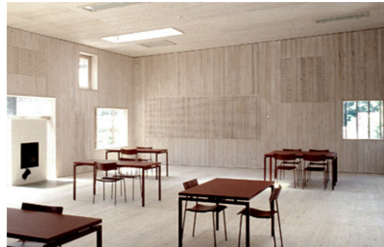
Ill. 123 - Sound proof panels in wood, village hall in Holbæk, BBP Arkitekter
