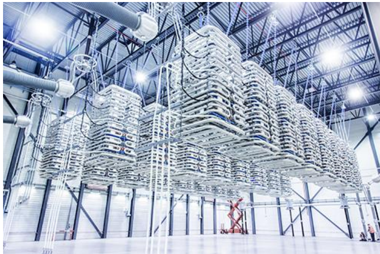
Figure 1.4: Skagerrak 4 converter station [11].
