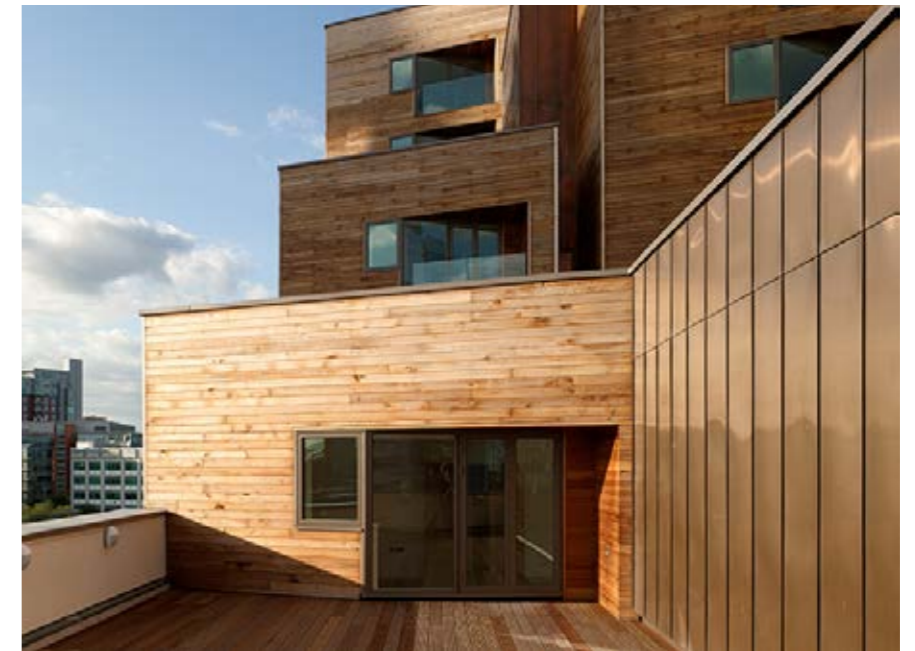
Illustration 156. Wooden elements together with copper plates seen in Watermans Place, Leeds (C) Dennis Gilbert.
