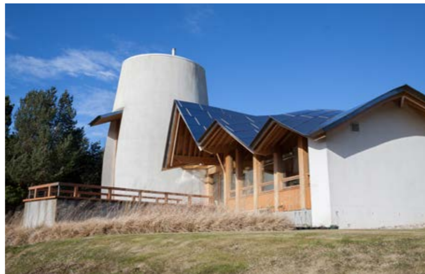
Illustration 102. The outdoor covering of the roof at Maggie's Dundee
