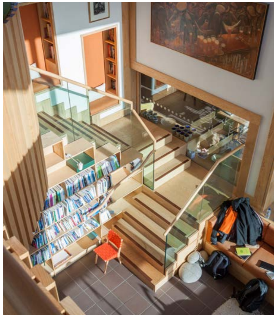
Illustration 77. Maggies in Newcastle. Connection between the stairs and the pockets in the wall.
