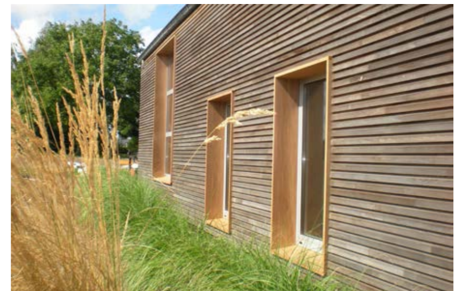
Illustration 157. Correlation between the window frames and the cedar siding. This siding type is called Free-Willy due to its cross section. Found on houtluyten.be
