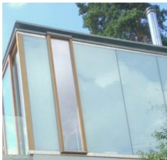
Ill. 131, Example of regular glazing together with aerogel glazing
