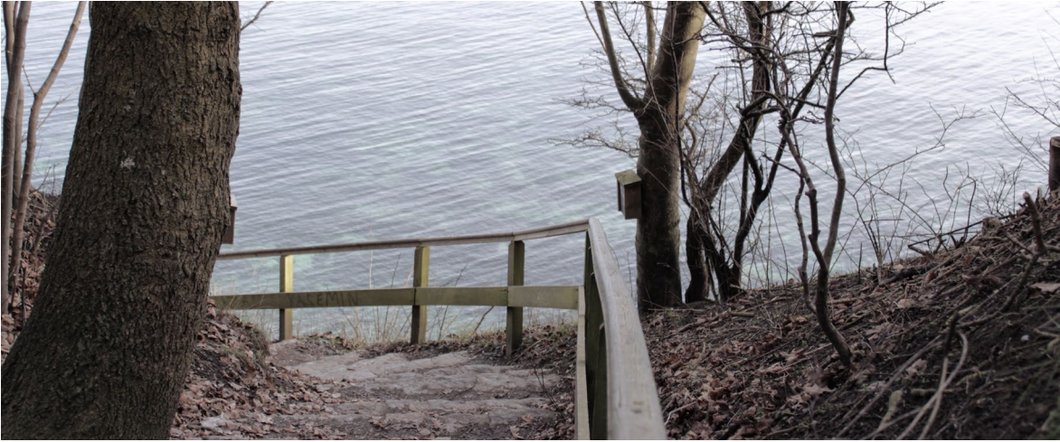
Ill 38a, View when going down to the staircase
