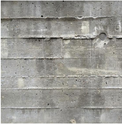
Ill. 90c, Concrete Wood boards form work
