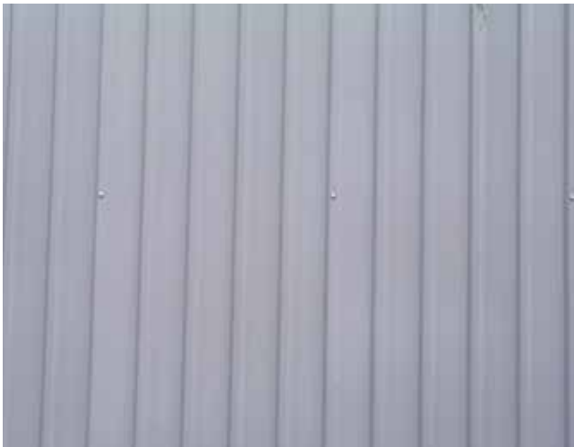
Fig 31.5: Zinc cladding with standing seam [mayang, 2015]
