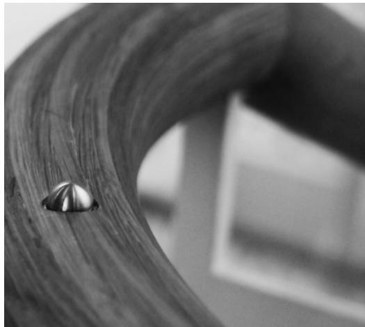
ill. 4.6 :: tactile marking of railing :: Handicaporganisationernes Hus :: Tåstrup
