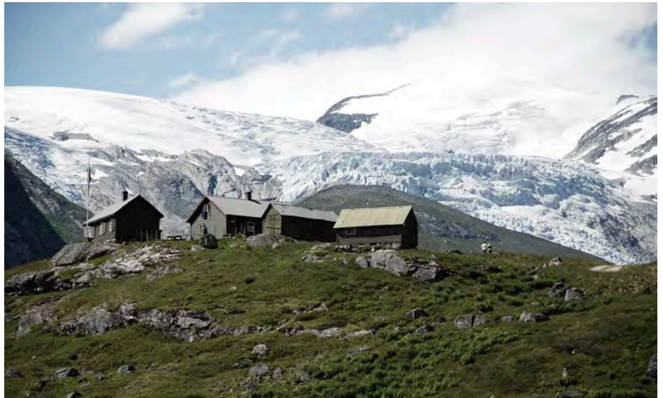
Ill. 1.12: The former Tungestølen complex
