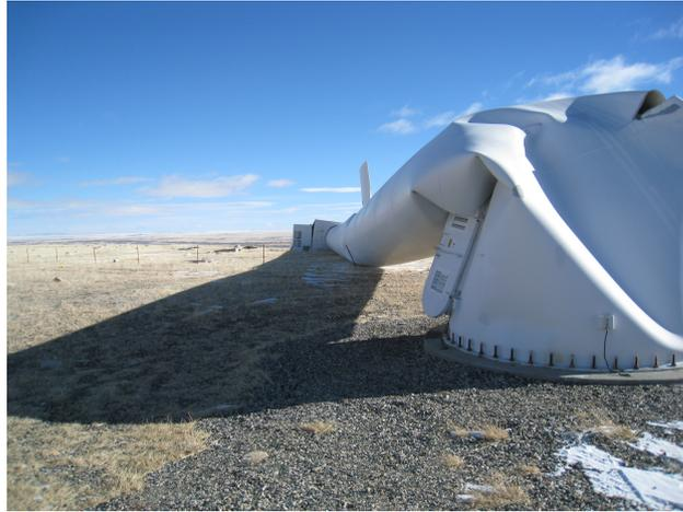
**Figure 1.1.** Dramatic collapse of a wind turbine tower at a wind energy facility, Arlington, Wyoming, [Brome, 2010]
