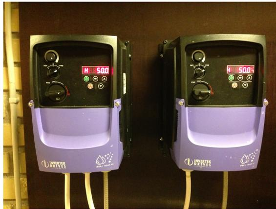
*Figure E.1.* Frequency converters used to control supply and extract flow.
