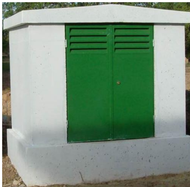
Figure 5.7 - Doghouse for air release valve
