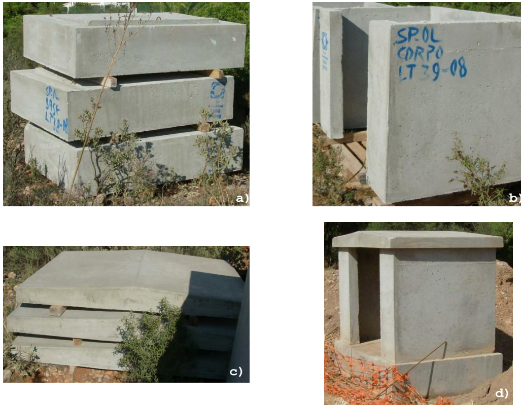
Figure 5.34 - Doghouse's air release valve: a) base, b) wall, c) cover and d) the completed element.
