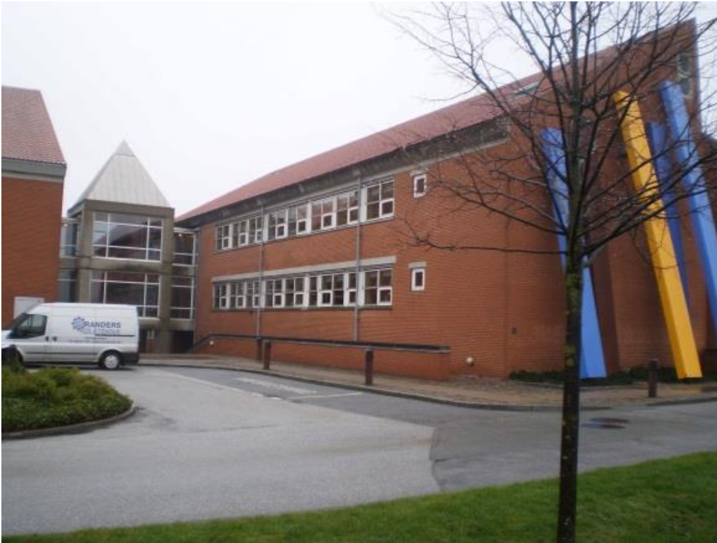
Figure 9: Building of Climate and Energy Department etc.
