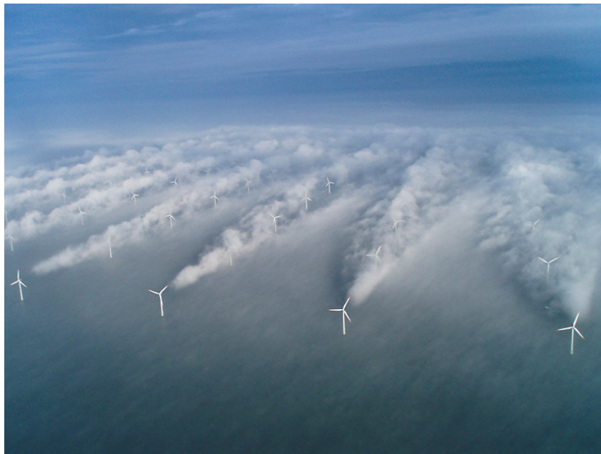
Figure 6.7. The wake effect at Horns Rev 1 [Aeolus, 2014]. Photo by Christian Steiness.
