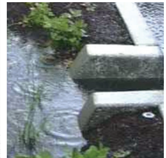
Ill. 134: Inspiration, leading water away from parking area
