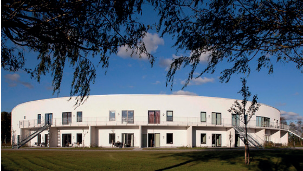
Ill. 60: Enghuset. Entrances, private terraces and gallery.
