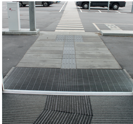
Ill. 18: Shift in flooring helps navigation for mentally restrained and people with visually impairment.
