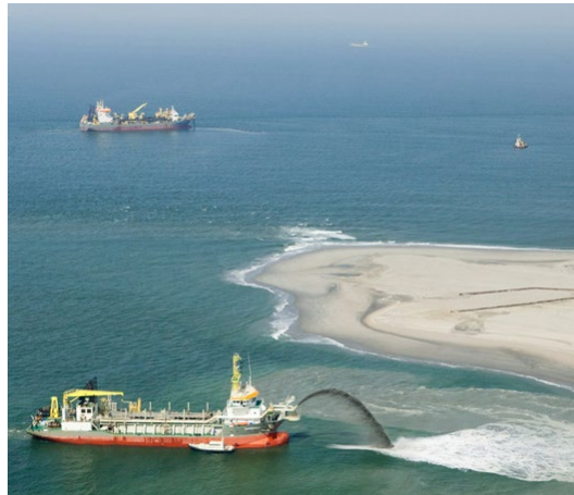
III. 72: Creating artificial island/peninsula by using the sand from the water bottom.
