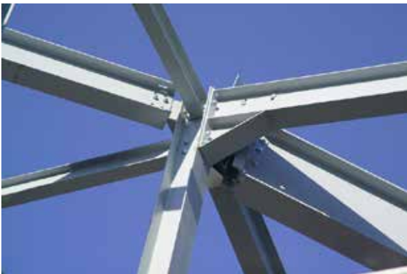
III 115 Example of steel column and steel beams
