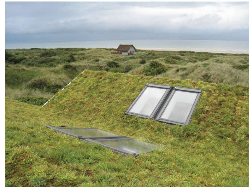
ill. 105 example of sedum roof with integrated skylight windows.
