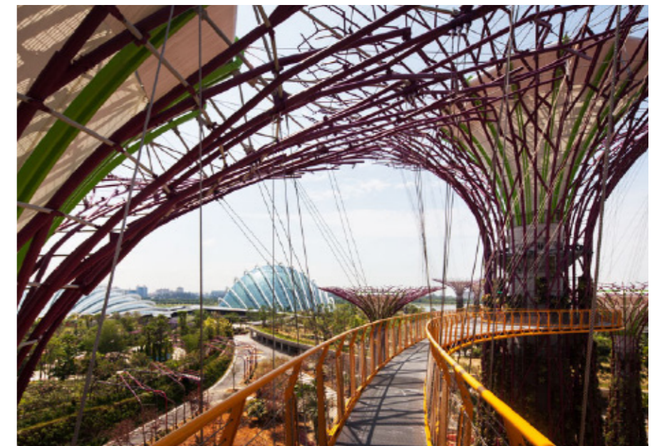
III. 90 // Walkway connecting the volumes.
