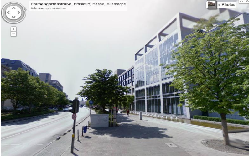
Figure 4-1 South facade of the building Ostarkade (Google Maps s.d.)
