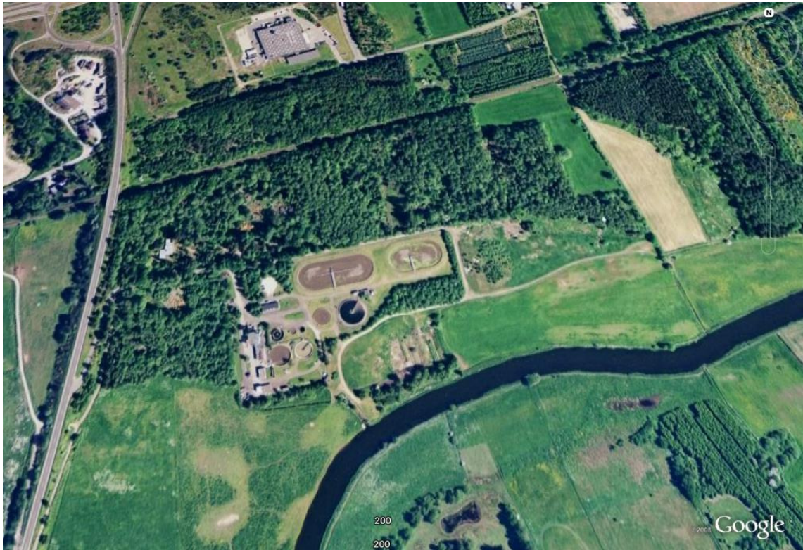
Figure 38. Bird's-eye view of Bjerringbro WWTP [8]
