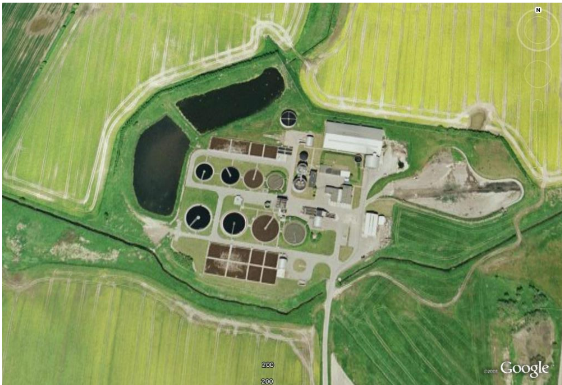
Figure 37. Bird's-eye view of Hjørring WWTP [8]
