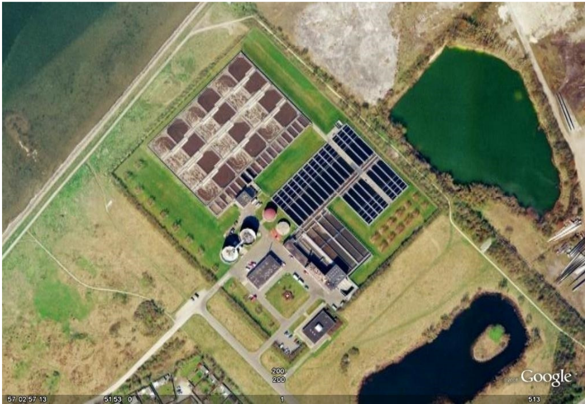
Figure 36. Bird's-eye view of Aalborg West WWTP [8]
