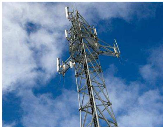
Figure 4-9: shows how the telecommunication companies cover all directions by putting more antennas on one BTS (mobilsiden.dk)<sup>25</sup>
