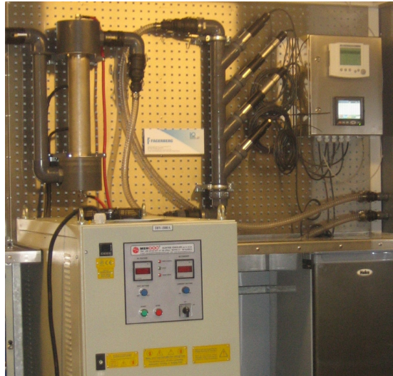
Figure 32: Electrochemical reactor placed above the installed power supply. The inline measuring cells for conductivity, ORP, pH, and DO are placed to the right.
