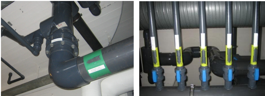
Figure 65: Left: the last meter of the main pipe before it splits up into smaller pipes. Right: the in- and outlets to UV, chlorination, and heat exchanger placed on the main pipe just before the pipe splits up.
