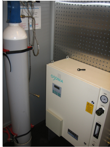
Figure 10: OZAT CFS-2G ozone generator from Ozonia and the installation in the test trailer.
