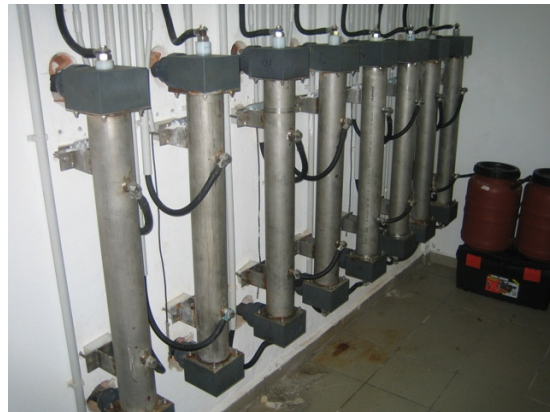
Figure 16: Photos from three different Watersafe swimming pool installations in Crete and 8 parallel operated Watersafe reactors from a waste water treatment plant.
