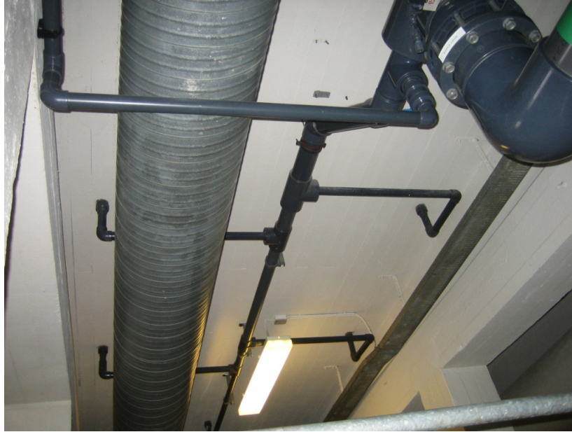
Figure 62: The main pipe with the treated water is divided into 6 separate inlets in the swimming pool. The photo is taken from underneath the pool.
