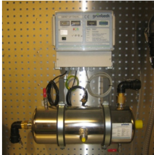
Figure 11: The installation of the UV disinfection system in the test trailer.
