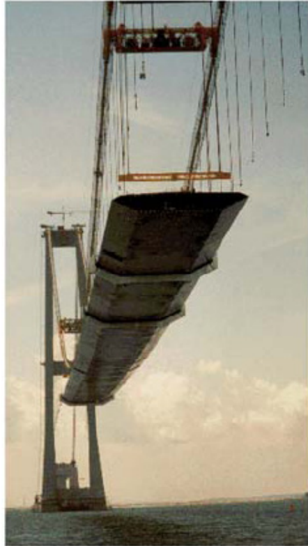
Figure 15: Illustration of the Great Belt Bridge with 249 meters of erected bridge deck. [Frandsen 2003]
