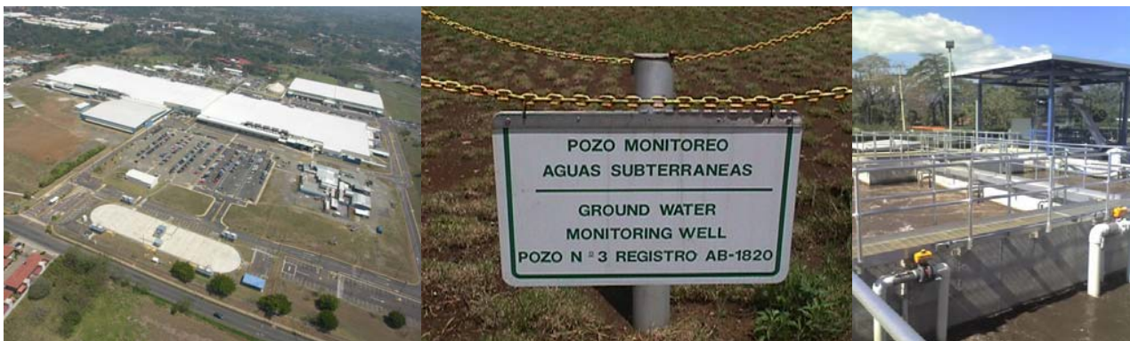
Figure 31 – (From left) Intel, aerial view; Groundwater monitoring well; Wastewater treatment system (Intel photos).
