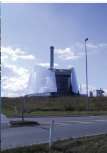
Thermal power station
